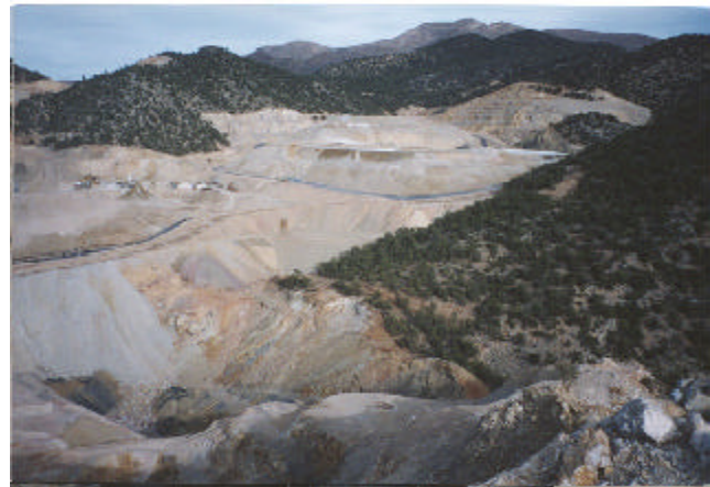
Figure 1.13: Heap leach operation prior to grading. Goldstrike Mine.
