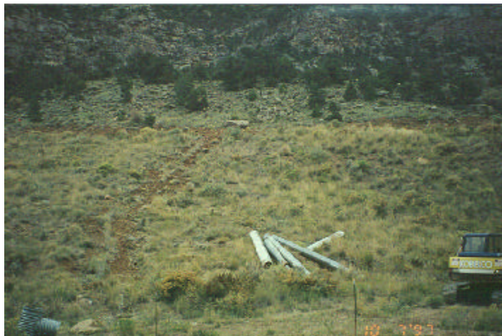
Figure 10.3: Slope drain was removed after vegetation was established. Horse Canyon Mine.
