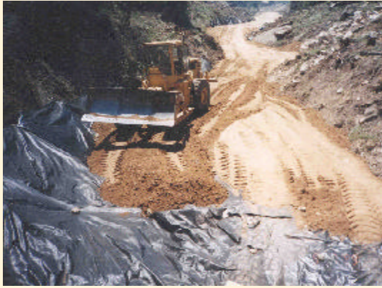
Figure 3.14: Fill material is placed on the geotextile mat. West Ridge Mine.
