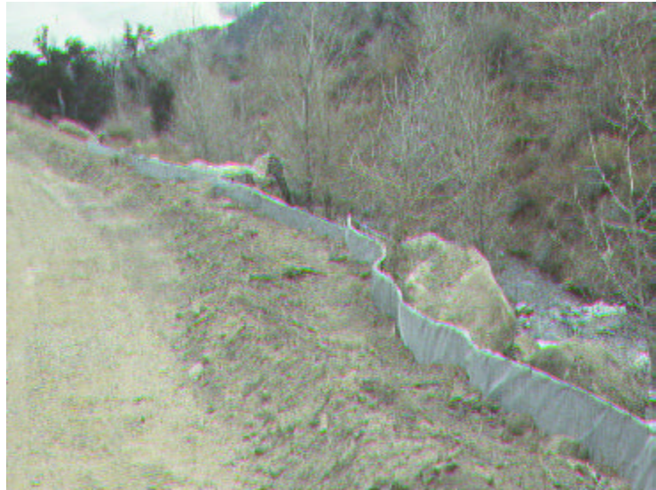
Figure 8.1: The silt fence is notched in a small drainage situation.
