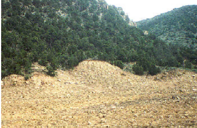
Figure 1.6: Minor drainages and ridge lines should be continued from the undisturbed into the disturbed area. Sunnyside Mine.
