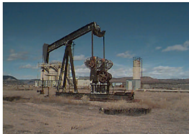
Figure 1.19: Oil well production site. Altamont - Bluebell Field Marker.
