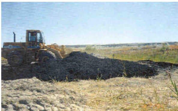
Figure 3.22: Biosolids additions to tailings. Kennecott Tailings Facilities.
