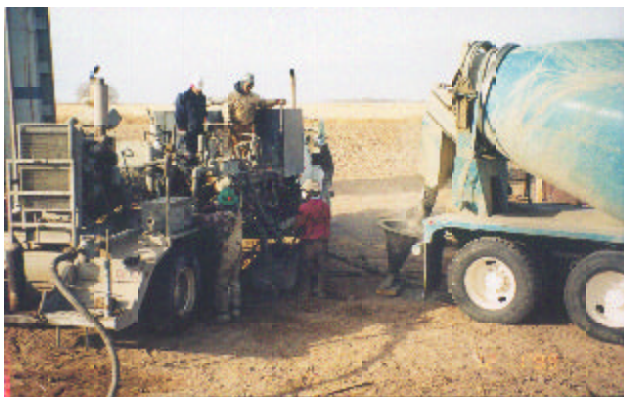
Figure 1.17: A well is plugged after operations have ceased.
