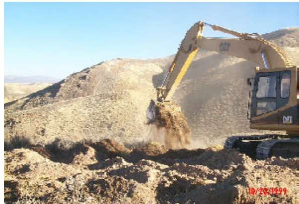
Figure 3.17: Extreme surface roughening breaks up compacted layers. Crawford Mine.
