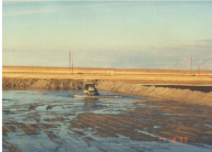
Figure 1,15: Tailings embankment construction. Kennecott Tailings Facilities.
