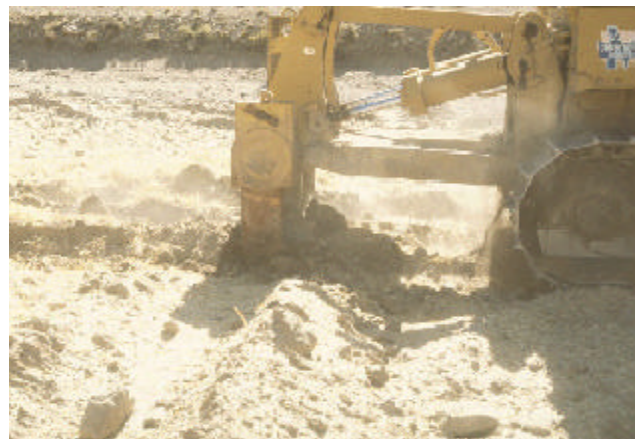
Figure 3.19: Deep ripping breaks up compact soil. Summit #1 Mine.
