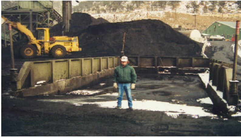
Figure 14.2: A temporary sediment trap near a washdown bay should be easily accessible for clean out by heavy equipment. SUFCO Mine.
