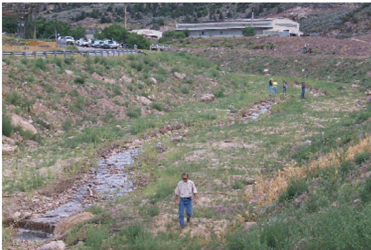
Figure 2.1: A road on the left and a railroad on the right of this channel dictated the channel design. Sunnyside Mine.
