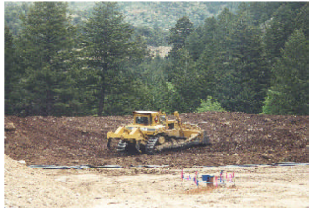
Figure 3.11: Topsoil pile construction. West Ridge Mine.
