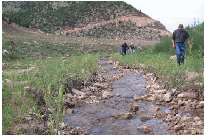
Figure 2.2: The channel was designed to allow water flow over the adjacent flood plain during high flows. Sunnyside Mine.
