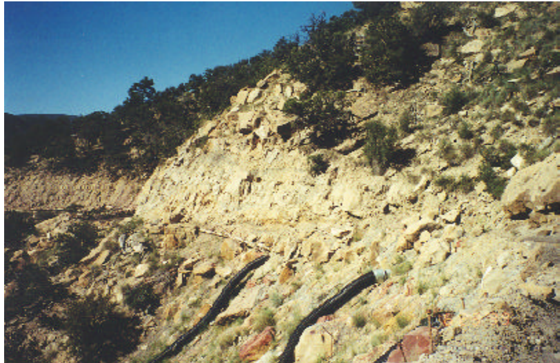
Figure 3.31: Flexible plastic culverts are attached to the ends of metal culverts conveying water collected on the road over the fill slopes. Bear Canyon Mine.
