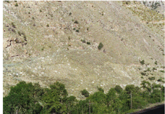
Figure 1.9: Both photos show reclaimed slopes. The left photo shows irregular topography, scattered boulders, and a patchy vegetation pattern that help the slope blend with its surroundings. (UP&L Carbon Plant) However, none of the same attributes are present in the photo to the right, causing the slope to contrast sharply with its natural surroundings. (Royal Coal Pile).
