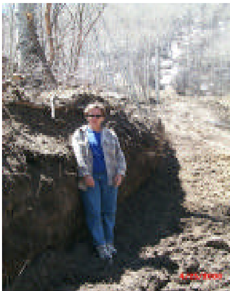
Figure 3.30: Uncontrolled water flow resulted in excessive grading on this road used for logging Carbon Co. activities.
