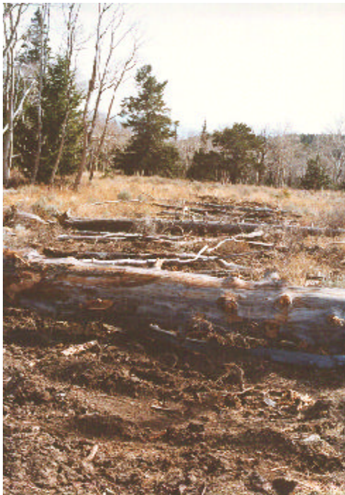
Figure 3.2: A roughened surface and slash mulch laid across this reclaimed exploration road prevents off-road vehicle access. Deer Creek Mine Exploration.
