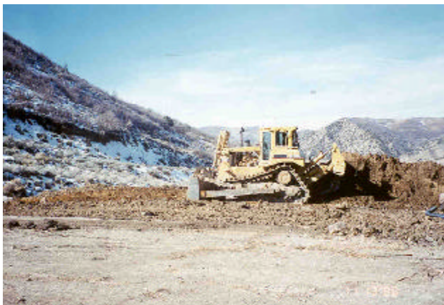
Figure 3.16: Use track equipment to reduce compaction. Summit #1 Mine.
