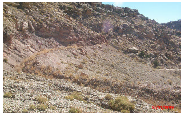
Figure 1.5: Diversion at top of slope during mining phase will direct water away from the slope. Failure to maintain the diversion will result in breaching and failure making these structures unsuitable for the reclamation phase. Hidden Valley Mine.
