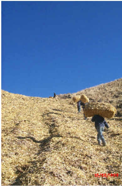
Figure 3.4: Straw is hand carried and spread in rough terrain. Crawford Mountains Phosphate Mines.
