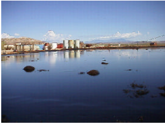
Figure 1.20: E&P waste facility. San Juan County.
