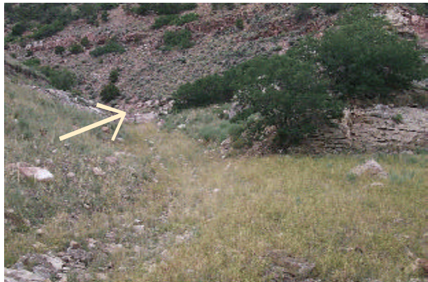
Figure 2.9: A defined ledge was excavated to allow adjacent concentrated flow to enter the drainage area in a controlled manner. Caste Gate Mine.
