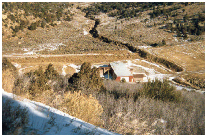
Figure 2.5: Entrenched channel with no developed floodplain. Knight Mine.
