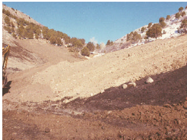
Figure 3.27: Acidic mine waste burial site. Boyer mine.
