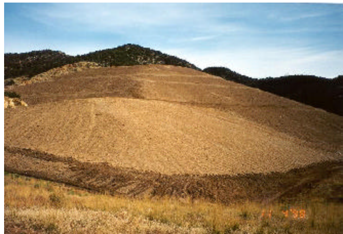
Figure 3.20: Terraces are used to reduce slope length on these reclaimed mine dumps. Goldstrike Mine.
