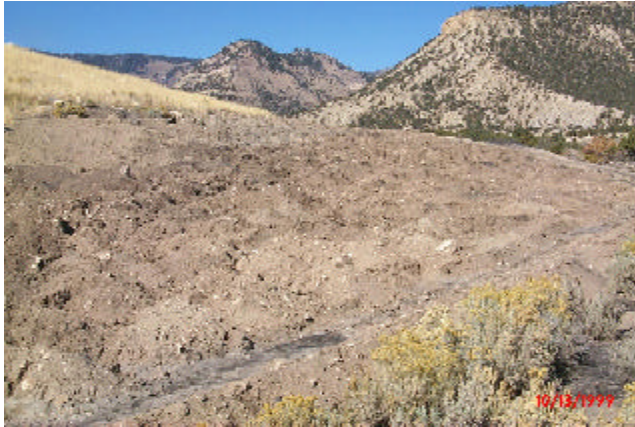
Figure 3.18: The soil surface is roughened, seeded and then hydromulched. Sunnyside Mine.
