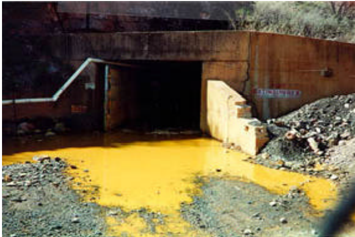
Figure 3.25: Typical acid mine drainage.
