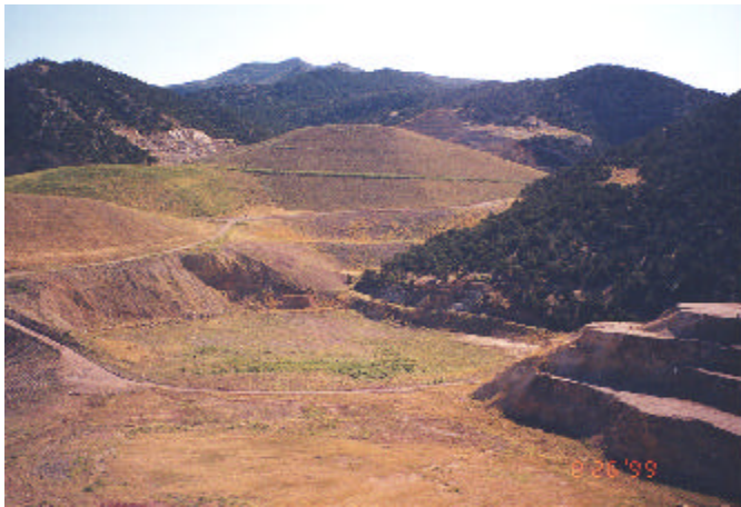
Figure 1.14: Heap leach operation after grading. Pits are backfilled and leach pads reshaped to blend into surrounding topography. Goldstrike Mine.
